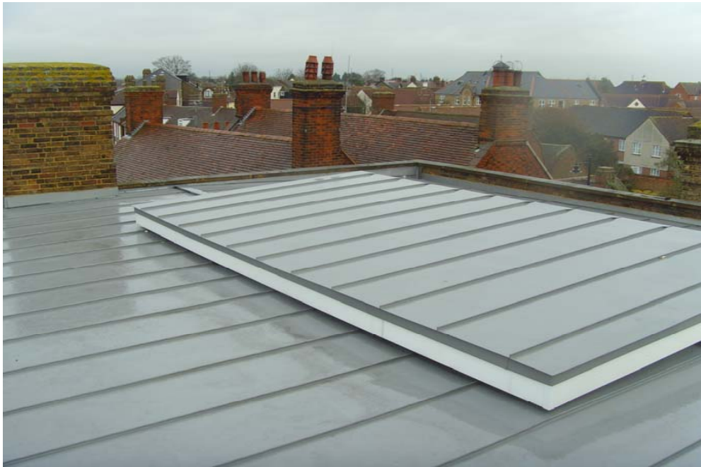
Roof now completely finished and covered - NOT with lead! Pictures taken January 2011 -after the snow had melted!
