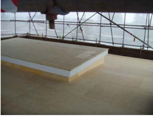
Roof planked, new 'roof light' - lower, lighter, and better insulated
