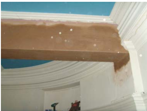
Cornices ready for fixing
