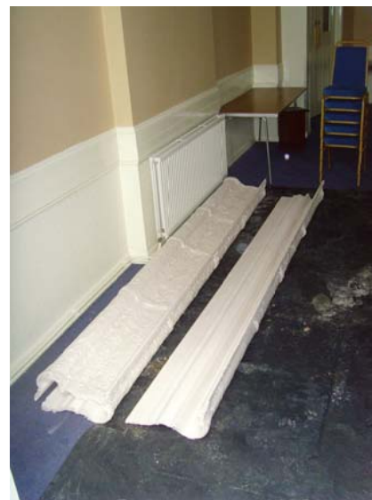
Cornices ready for fixing
