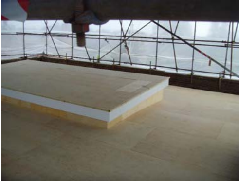
Roof planked, new 'roof light' - lower, lighter, and better insulated
