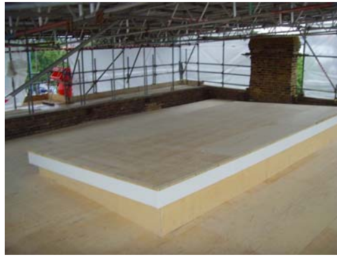
Roof planked, new 'roof light' - lower, lighter, and better insulated
