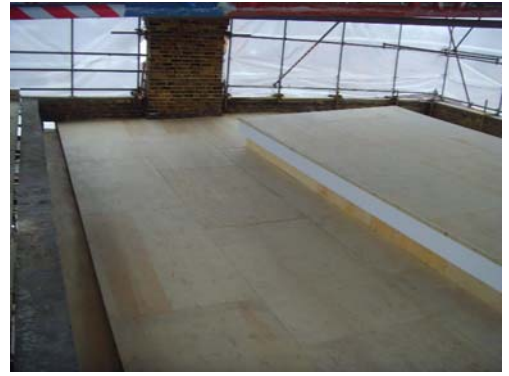
Roof planked, new 'roof light' - lower, lighter, and better insulated
